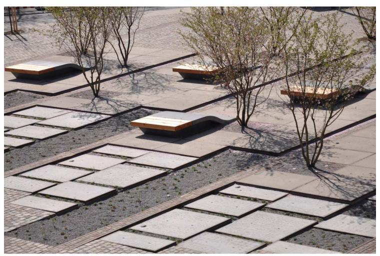
Low-maintenance beautiful planters are actually cleansing and infiltration points for a large subsurface gravel trench, from where the rainwater can recharge the groundwater table. Using this innovative, load-bearing filter medium reduces the hydraulic overload on the sewer system. No rainwater is fed into the sewer system; instead the groundwater table is recharged.
