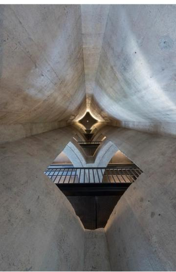
The new concrete sleeves created a stable composite structure 420 mm thick and provided a cutting guide for removing portions of the old silos. The existing tubes were pared back to reveal the curved geometries of the 4,600-cubic-metre atrium. The cut edges were polished to give a mirrored
