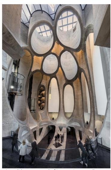
Though the concrete building looks like a single structure, it is composed of two parts: a grading tower and 42 tall, cellular silos.
