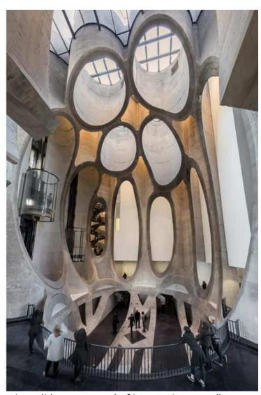
Though the concrete building looks like a single structure, it is composed of two parts: a grading tower and 42 tall, cellular silos.
