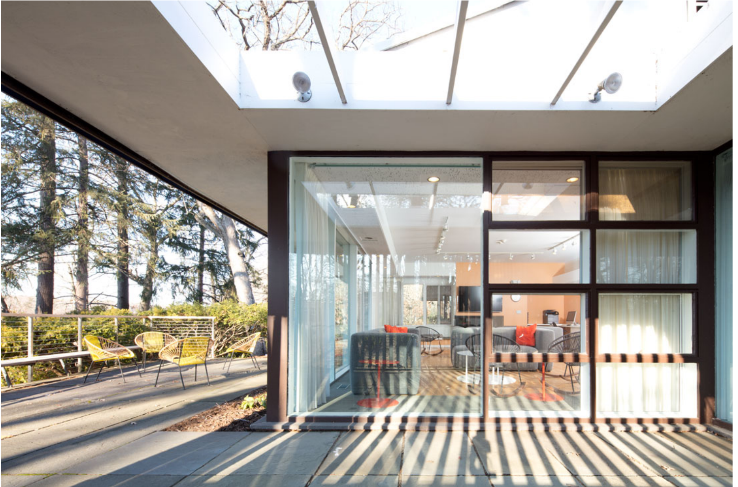
View of renovated outdoor terrace and social lounge. (Studio Luz Architects, Terrace, Acorns House, Wellesley, Massachusetts, 2016. Photo by John Horner.)
