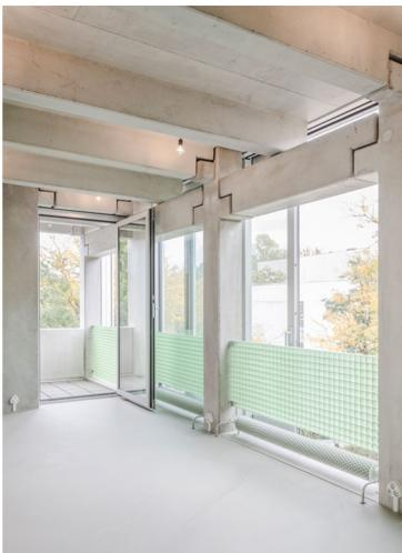
A curtain wall consisting of large-scale standard sliding glass doors makes up the eastern and western façades. It allows for the interior to be opened up to its surroundings during the spring and
