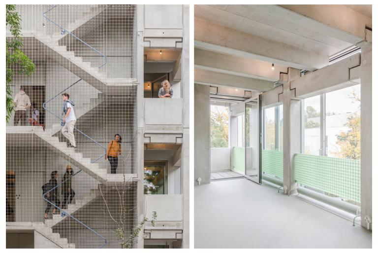
A curtain wall consisting of large-scale standard sliding glass doors makes up the eastern and western façades. It allows for the interior to be opened up to its surroundings during the spring and
