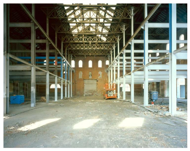
The steel column and beam structure and the brick outer shell are cleared of any superfluous additives.
