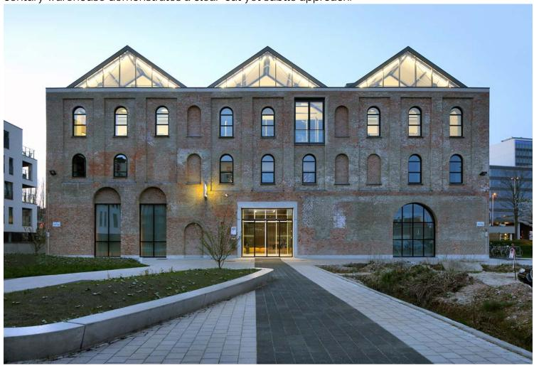
The administrative headquarters of the East Flemish home care organization was constructed without interfering with the original three-aisled structure. The interventions were designed as a new subordinate layer within the dominant structure of this typical Mancunian factory architecture.
