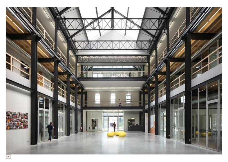
The steel column and beam structure and the brick outer shell are cleared of any superfluous additives.
