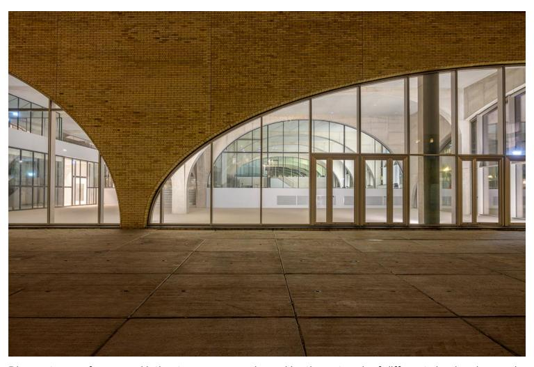
Diverse types of open and intimate spaces are shaped by the network of different sized arches and differences in floor heights. Additionally, the arches are a visual and structural transition between the basement car park, with its wide spans, and the 150 dwellings above. Broad arches in the façade frame and highlight the cultural activities within, with the largest arches positioned at the corner as an inviting gesture from this prominent address.
