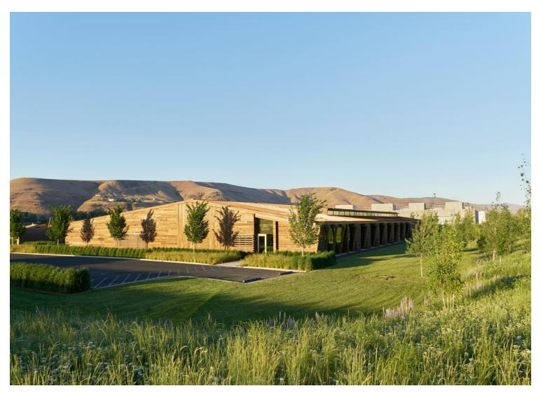
The L-shaped building is nested into the landscape through the use of board-formed concrete site walls and earthen berms that wrap the perimeter to form a central, landscaped courtyard. Soil excavated for foundation work was repurposed for the perimeter berms, eliminating the need to remove it or add more.
