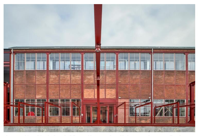
The Assembly Hall is a heritage building, and in connection with the conversion, C.F. Møller also contributed an analysis of the conservation value of the hall. This value relates, among other things, to the hall's 200-meter-long building volume, the façade's red steel grating structure, infilled with panels of red brick, and the characteristic gable motif, expressed in the hall's curved roof and prism-shaped skylights.
