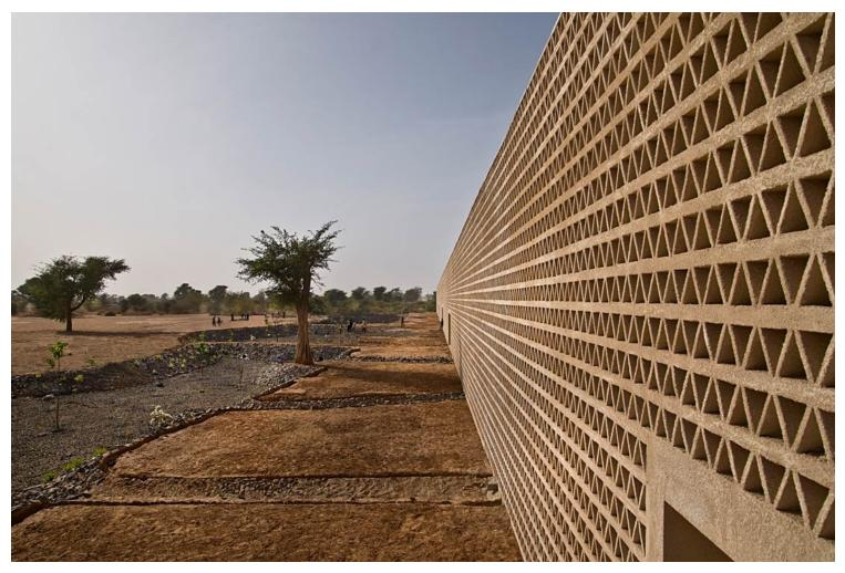
The combination of the double roof and the double-skin façade, with 1-meter and 3-meter cavities respectively, makes it possible to create a breeze: the heat concentrated on the outer skin of the façade ends up flowing under the roof, pushed along by its inclination. This system allows for a high percentage of outside heat to be dissipated while at the same time generating a constant flow of air through the cavity of the building's envelope.
