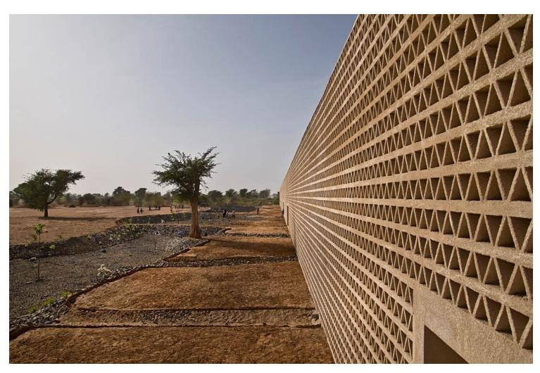
The combination of the double roof and the double-skin façade, with 1-meter and 3-meter cavities respectively, makes it possible to create a breeze: the heat concentrated on the outer skin of the façade ends up flowing under the roof, pushed along by its inclination. This system allows for a high percentage of outside heat to be dissipated while at the same time generating a constant flow of air through the cavity of the building's envelope.
