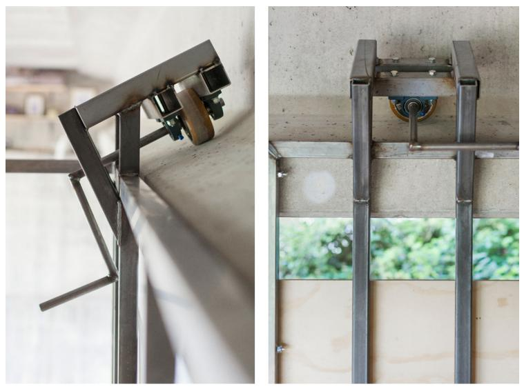
In the execution, we made use of the existing beams under the bridge using them as rails over which a carriage rolls (disassemblable metallic structure). At the end of its path, it links with the furniture creating a useful homey space.
