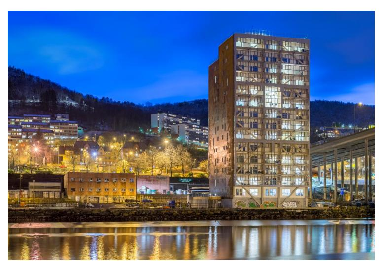
The main principle of the building is independent modular units with their own walls, roofs, ceilings and roof construction, stacked between the main glulam framework. All gaps are closed with insulation, and the building is coated with an outer shell to weather protect all the individual parts and the gaps between them.
