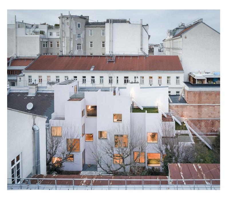
The entire built-up area is compensated by retention roofs and intensively planted passages. In order to avoid an entirely uni-directional orientation of the elongated building, it was divided into a grid of 20 square fields with projections and recesses in plan and varying heights in section that
