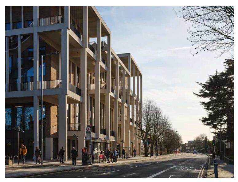
While the building feels permeable and transparent, environmental control is achieved through the use of 'colonnade' and 'ambulatory' elements. Recessed on three sides to form gardens and colonnades, the façades are open and transparent at the lower levels becoming more solid at the upper levels where shading is required. This colonnade plays a central civic role and establishes the important presence of this new University building within the public realm.
