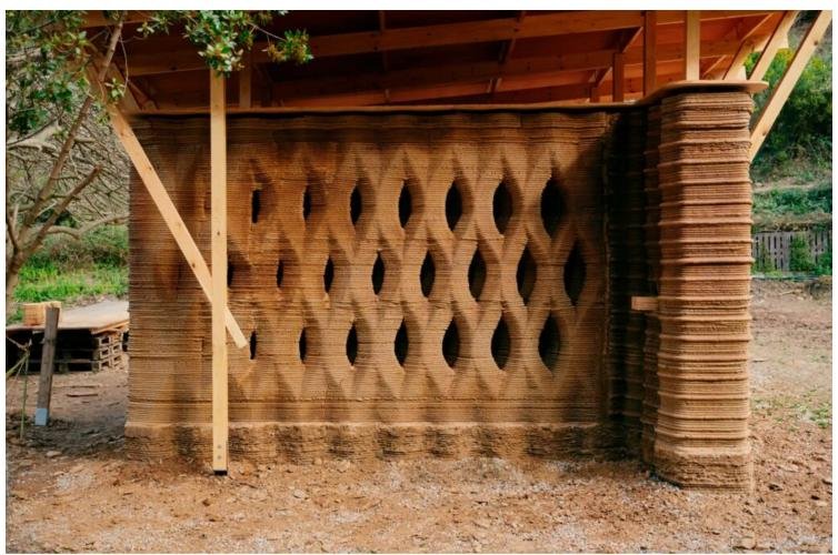
TOVA incorporates a variety of sustainable features, such as walls designed with air cavities for insulation and a compact, expandable structure to maximise outdoor living space. The construction process generates zero waste and utilises a unique mixture of local materials to ensure environmental sustainability.
