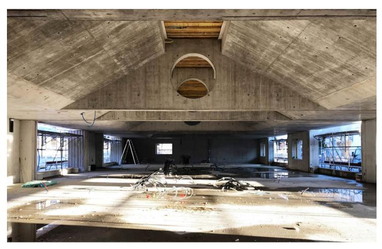
The concrete beams in combination with the wooden, non-load-bearing fixtures divide the interior into three kindergarten compartments, which are connected by large sliding doors. Circular openings in the concrete beams allow visual connections between the main rooms and the cozy, skylit mezzanines between the beams.
