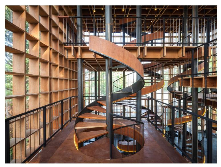
All five spiral staircases were designed not only for circulations to fit into limited spaces but also to serve as structural supports. Furthermore, the usual experience of scale and the amount of spiral stairs have been sculpted to form an unfamiliar new space, arousing in visitors the sense of the abstract.
