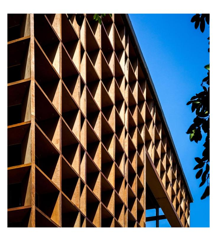
The waffle walls can be a light filter to help cool down the interior atmosphere. Boonserm Premthada
