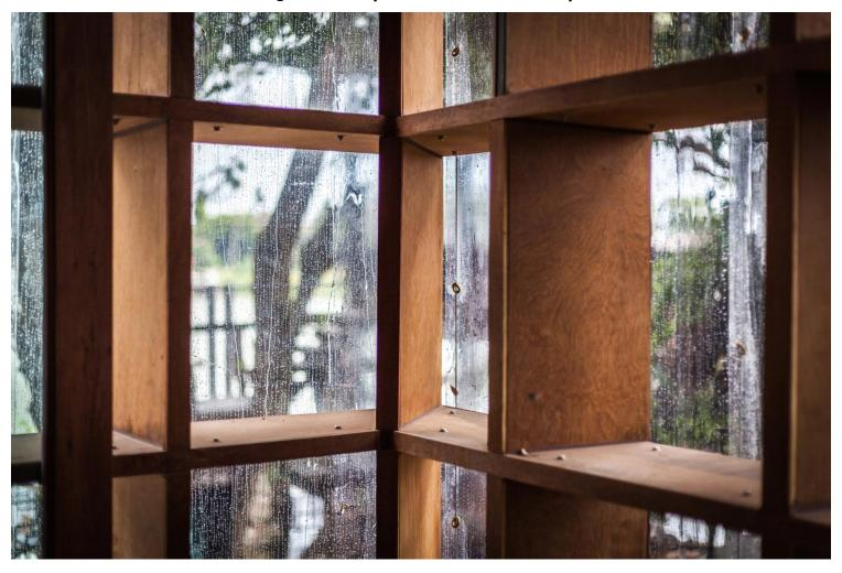
The building is protected from rain and humidity by coating the plywood with resin and covering the building with 1 millimeter thick PVC sheets. Boonserm Premthada
