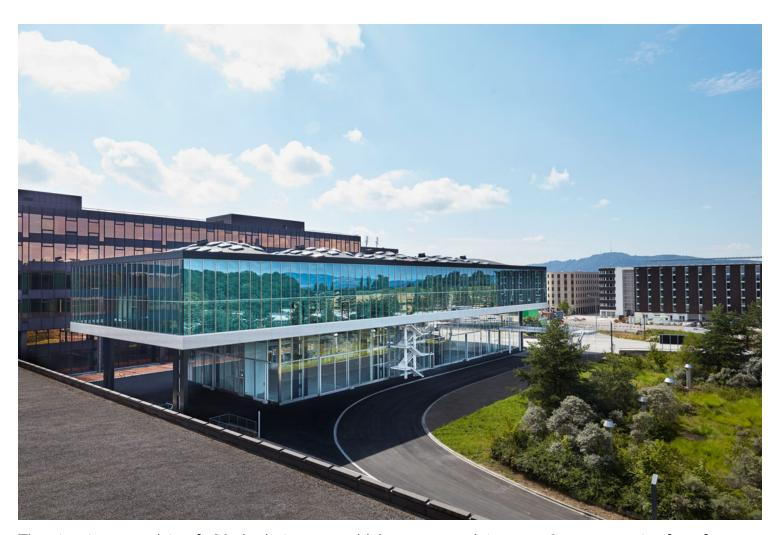
The structure consists of 168 single trusses, which are woven into a 2,308 square meter free-form roof design. As such, an integrated digital planning process connects design, structural analysis and the generation of fabrication data. Based on this data, a robot-based assembly process joining 48,624 timber slats to individually formed trussed beams allows an efficient fabrication of the complex roof geometry.
