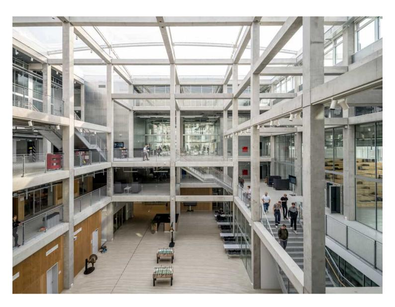
The interior construction has exposed bare concrete surfaces and the building's floors have a robust surface that can withstand heavy use on the ground floor and in the workshops. The interior walls between the atrium and the teaching rooms have sections of glass to ensure visibility and dialogue. Overall, the building has a simple and honest expression based on functionality and utilization.
