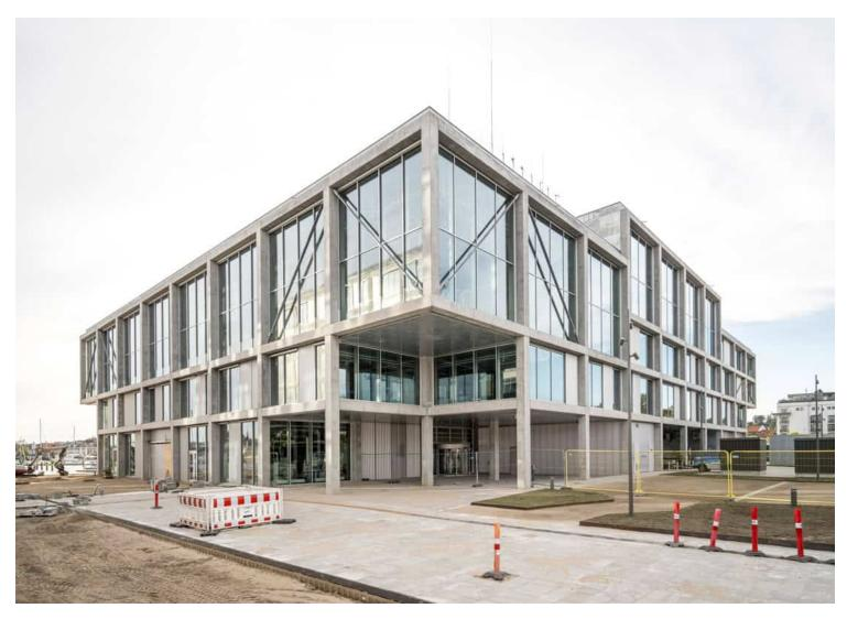
The architectural design is based on a modular construction grid that maximizes openness and flexibility in the physical framework of education. The construction is flexible and allows for reorganizing the layouts for workshops and teaching rooms without disturbing the load-bearing structure and logistics. The design provides a good spatial range, which can function for both larger classrooms as well as workshops, but can also be subdivided into smaller units for offices.
