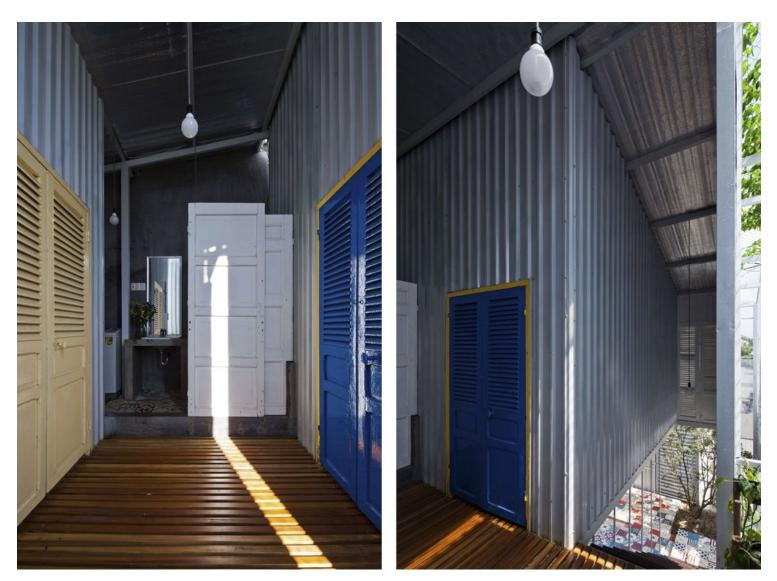
Without a doubt, using a steel structure not only makes the foundation requirements lighter, it also helps shorten the construction period, while saving on costs as well. The house frame is made up of 90x90 steel columns and 30x30 steel beams connecting to metal sheets. The structure is then covered or filled in by plants so, from a distance, the house looks like a green box. Among these "cool-metal" bars, the natural elements are defined.
