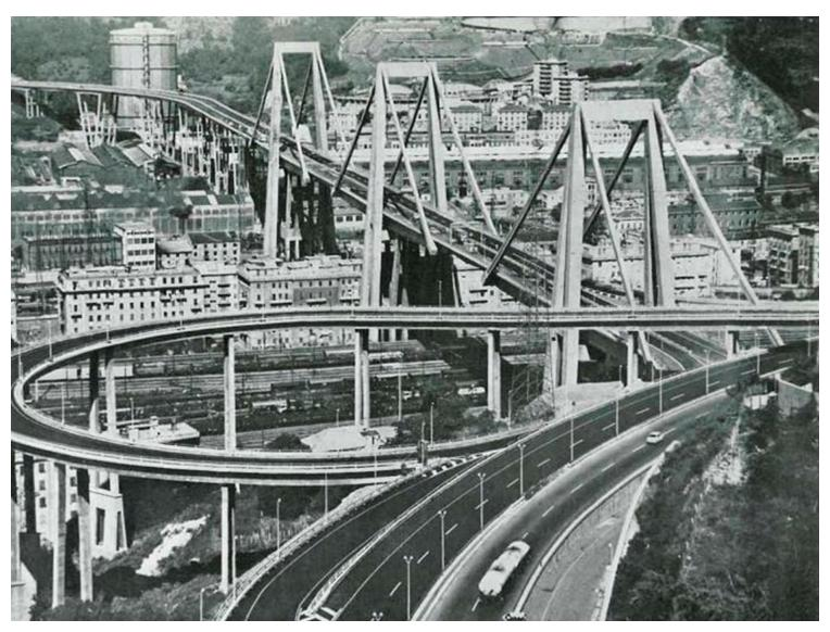
Built between 1963 and 1967 by the Italian company Condotte d'Acqua, the bridge had a length of 1.18 kilometers, a height of 45 meters and three large A-shaped concrete supports that reached 90 meters. The length of the main span was 210 meters.
