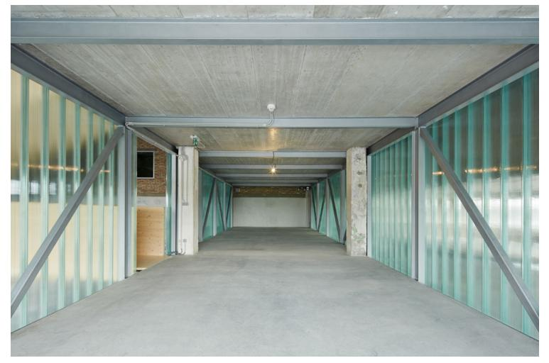
The rigid construction of the structural skeleton is complemented by transparent partitions in the new layout, soft timber infill panels, Profilit walls and exposed ducts. Three new floors for administration are created within the original concrete hoppers, which are made accessible from the central hall.
