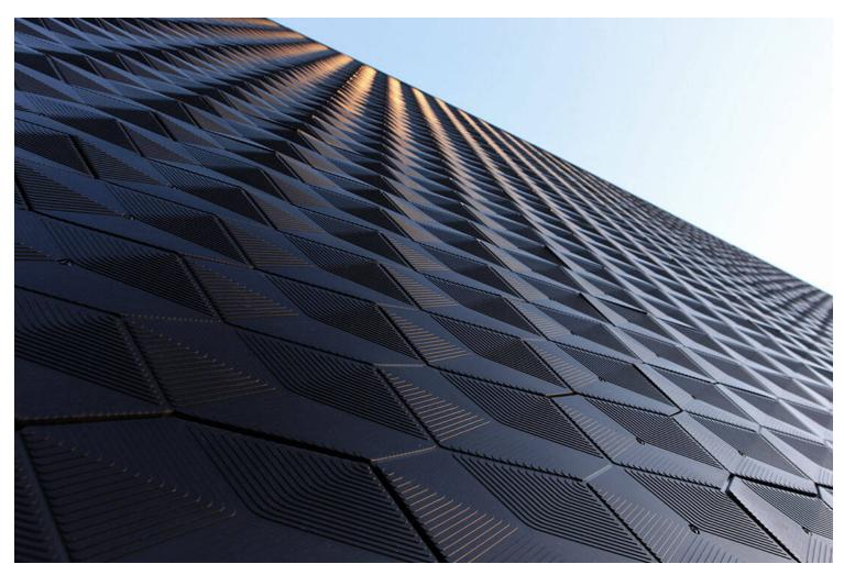
The product is a combination of Made of Air's proprietary functionalized biochar, the key carbon-negative element, and bio-based polymer binders. The result is granular materials that can be thermoformed using existing processes. In effect, this material is a permanent carbon sink that goes beyond reducing embodied emissions, providing the double benefit of carbon removal and avoided emissions. For the Audi application, 10 tons of CO2 have been sequestered from the atmosphere.
