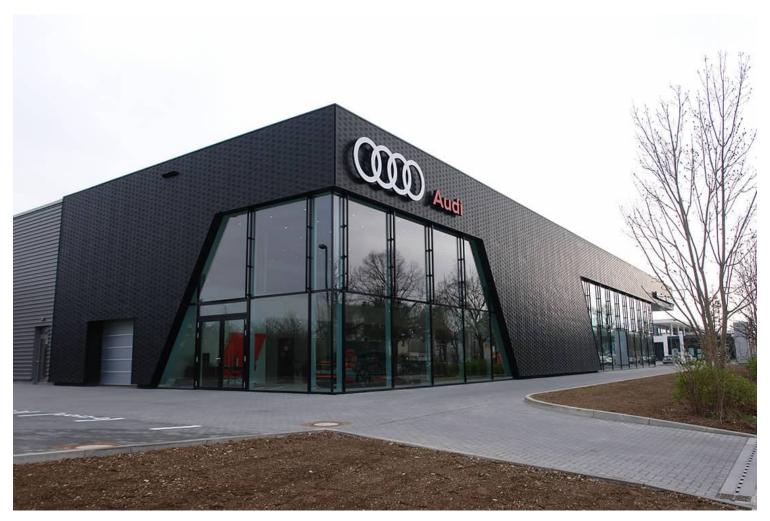
The brief was to create a cladding from a sustainable product to replace the typical aluminum that Audi used. Simultaneously, it was critical to keep to Audi's high-end and branded design while meeting product requirements. For the project ~600 square meters of product was produced following a co-development program.
