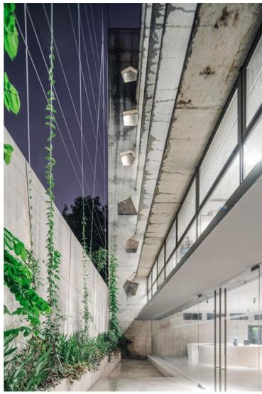
The mesh net on the entrance side and green façade cabling at the rear of the building provide passive shading and offer a sense of intimacy. At the back of the building, the open vertical space allows the site to generate its own light and ventilation, a soft filter from the nearby chaos.
