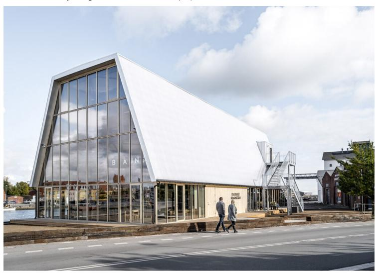
The Taphouse is built from just a few, sustainable materials that are not mixed as far as possible. This has reduced the volume of waste from the construction considerably, compared to similar constructions. The building is based on simple tectonic principles and is completed with mechanical joints only. All primary wall surfaces are without paint or grout. Wooden floors are laid using waste product from the nearby flooring manufacturer Junckers.
