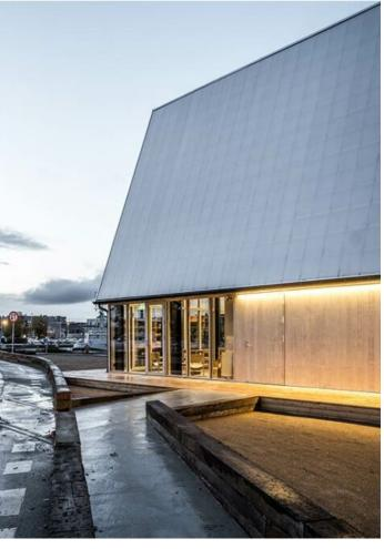
The large roof surfaces are made from click-joint polycarbonate, while wood façades are made from the CO2-neutral Accoya that is certified Cradle2Cradle Gold, FSC as well as the Danish eco-label Svanemaerket. The Taphouse is partly self-sufficient with electricity from solar panels, and natural ventilation reduces the need for mechanical ventilation.
