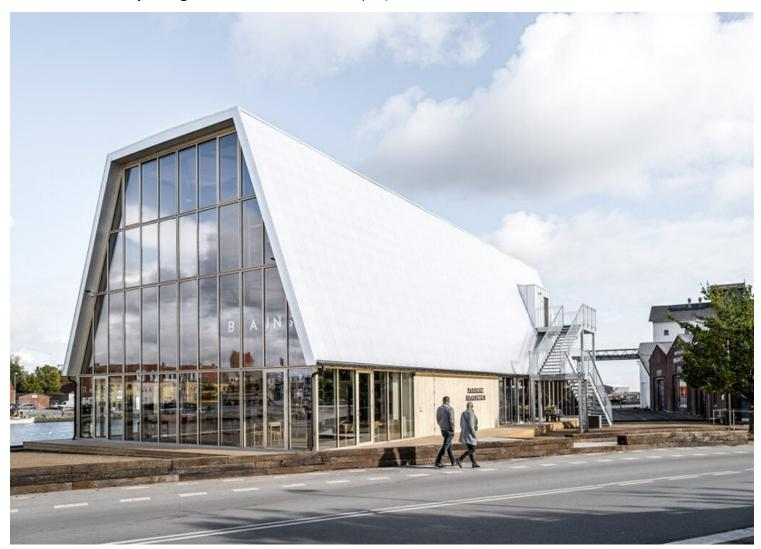
The Taphouse is built from just a few, sustainable materials that are not mixed as far as possible. This has reduced the volume of waste from the construction considerably, compared to similar constructions. The building is based on simple tectonic principles and is completed with mechanical joints only. All primary wall surfaces are without paint or grout. Wooden floors are laid using waste product from the nearby flooring manufacturer Junckers.
