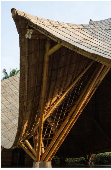
"The Arc operates like the ribs of a mammal's chest, stabilized by tensile membranes analogous to tendons and muscles between ribs. Biologically, these highly tensile microscopic tendons transfer forces from bone to bone. In The Arc, bamboo splits transfer forces from arch to arch."
