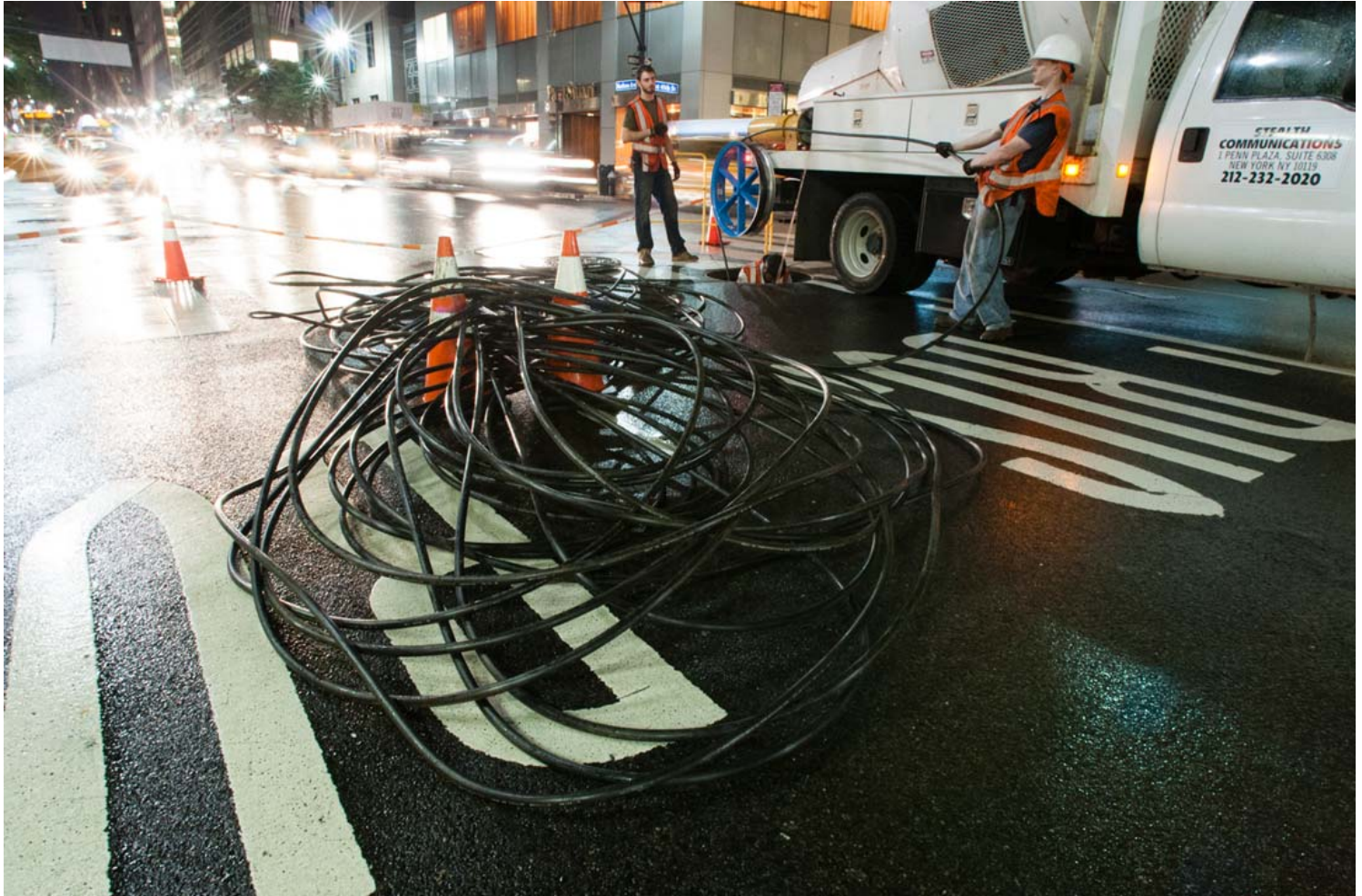
Crew installing fiber cable underneath the street. Photo by Stealth Communications.
