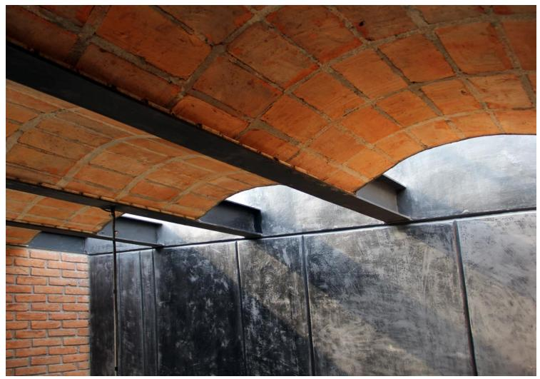
The technique of leaving the concrete and brick exposed provides a window into the development and design of the structures. For example, the brick vaults rest upon IPR beams at double height, supported by a wall of exposed concrete. The concept of a double-height space within the limitations of the property presented both a design challenge and an advantage, because it did not require the sacrifice of other spaces.
