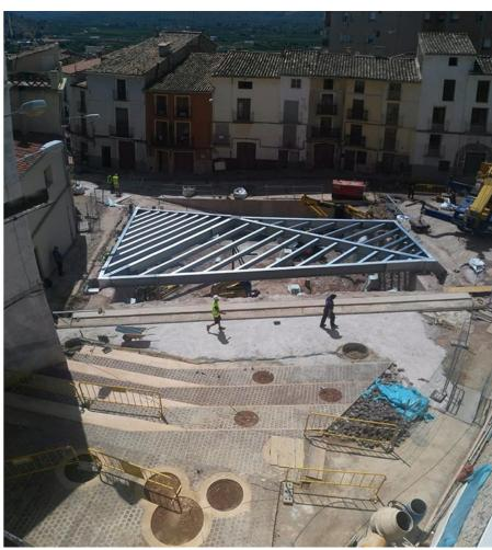
A smooth ramp connects to the lower space. A manual ceramic pavement is laid on the floor of the old pond, an interpretation of the compacted clay pavement found there. The pond recovers the memory of the water.
