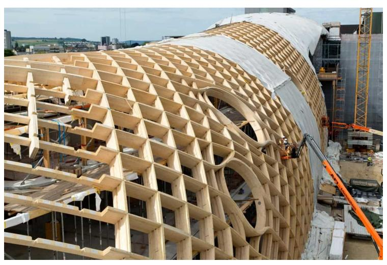
While the wooden structure was still being erected, the installation of around 2,800 honeycomb elements (timber grid shell), which make up most of the façade, began. Each element was meticulously tailored from up to 50 individual parts and adapted to its individual function and position. Three basic types of honeycomb can be distinguished: the opaque, the translucent and the transparent element.
