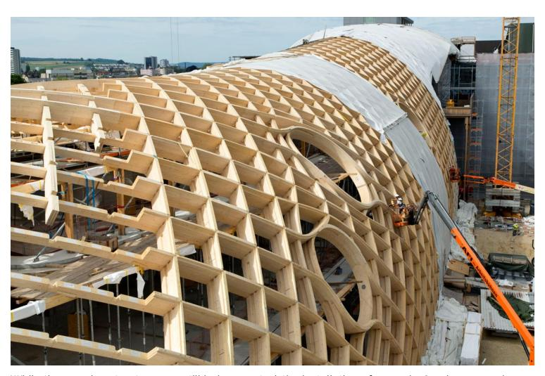
While the wooden structure was still being erected, the installation of around 2,800 honeycomb elements (timber grid shell), which make up most of the façade, began. Each element was meticulously tailored from up to 50 individual parts and adapted to its individual function and position. Three basic types of honeycomb can be distinguished: the opaque, the translucent and the transparent element.
