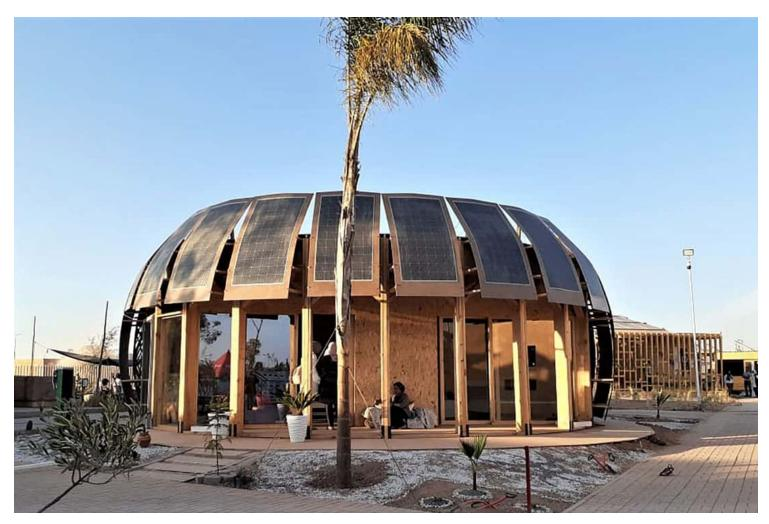
The modular, off-grid hemp home is inspired by the needs of remote regions like the Moroccan Central Rif. A spherical building skin made from a hemp fibre bio-composite integrates frameless
