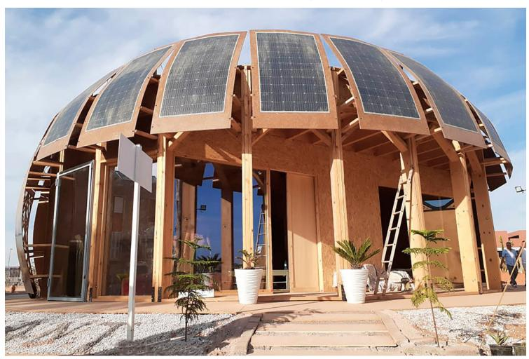
The project takes additional advantage of the aforementioned material qualities through a compact, aerodynamic design that minimizes exposure to the environment. A bioclimatic layout, inspired by the vernacular architecture of the region in question, functions with natural ventilation, a favourable orientation of the habitable spaces, and an optimised arrangement of openings. A high-end glassing completes the performance.
