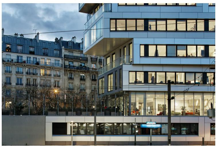
Two vertical circulation cores connect the upper floors with the ground level and the underground parking area. The office complexes are divided into two compartments of less than 800 m<sup>2</sup> in order to allow for natural ventilation. The surfaces can be divided according to a 2.70m framework, corresponding to the elements on the façade.
