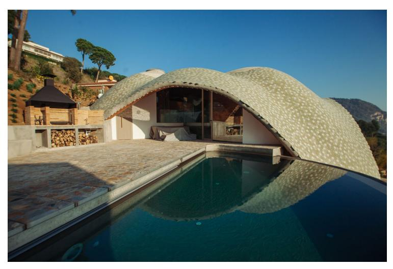
Our reinvention of the Catalan vault was rooted in advanced engineering using fiberglass, whereas the challenge facing the ceramists involved creating a tile that would be in harmony with the natural conditions of the site, since the core of this design is its integration.
