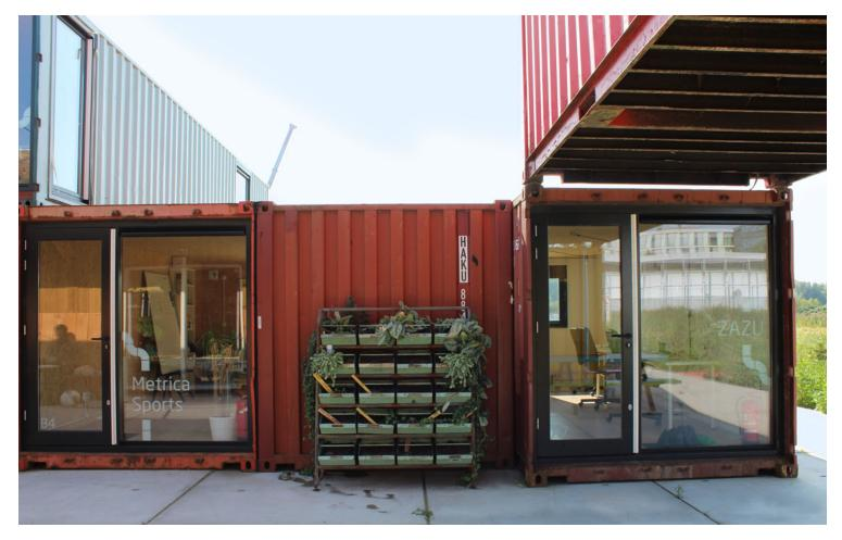
The shipping containers can be clad and placed in many different ways, which makes the shipping container quite an interesting architectural element for building quick and low-cost sculptural and temporary buildings.
