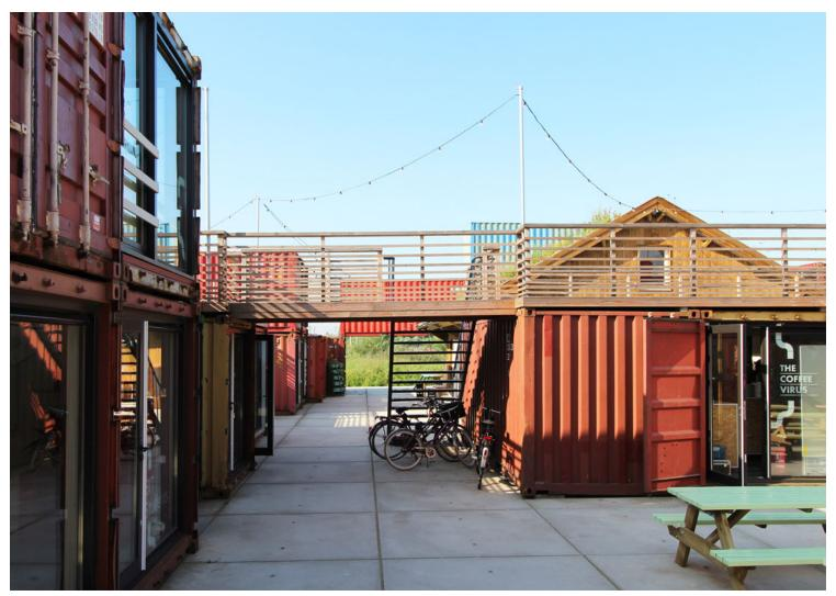
The dimensions of the upcycled containers (2.4 x 6 meters (a small 20 ft container)) are perfect for startups and provide an affordable and lockable office space. There are also connected 20 ft (4.8 x 6 meters) and 40 ft containers (4.8 x 12 meters) which can be used for scale-ups.
