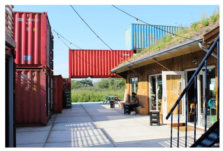
The containers have a high percentage of glazing in comparison to the floor area and are much brighter than "standard" offices. The spaces are very efficiently used; hallways and other traffic areas are outside the container, since most of the communal spaces are focused on the central square. The central square and its communal spaces serve as a big meeting point.
