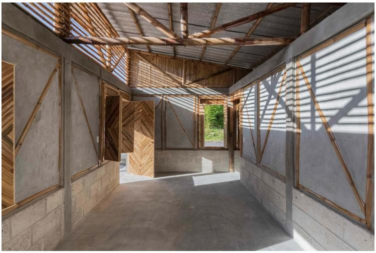
Once installed, the bamboo panels are coated with ixtle (local fabric used to make coffee sacks) and a thin layer of mortar. Once the base structure has been placed, the beams and subsequently the ecolam sheet are fixed. The latter is a product made from food-grade aluminum waste, which gives thermal, acoustic and antibacterial properties.
