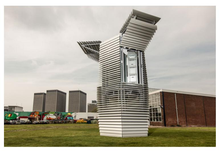
Roosegaarde and his team of experts have used patented ion technology to build the world's largest smog vacuum cleaner. The Smog Free Tower produces smog-free bubbles of public space, allowing people to breathe and experience clean air for free. The first 7-meter high Smog Free Tower cleans 30.000m3 of air per hour of ultra-fine smog, uses no more electricity than a water boiler, and runs on green energy.
