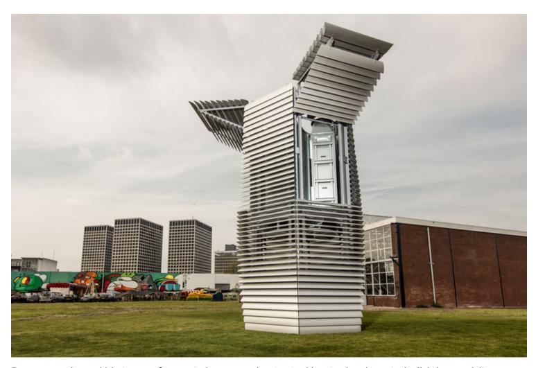
Roosegaarde and his team of experts have used patented ion technology to build the world's largest smog vacuum cleaner. The Smog Free Tower produces smog-free bubbles of public space, allowing people to breathe and experience clean air for free. The first 7-meter high Smog Free Tower cleans 30.000m3 of air per hour of ultra-fine smog, uses no more electricity than a water boiler, and runs on green energy.
