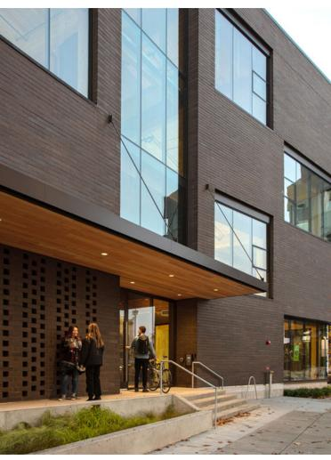
The wedge-shaped building features a new CLT structural system with an open ground-level commuter-oriented retail environment geared toward guests and tenants. The workspace above is wrapped in brick masonry with the building acting as an anchor for the Burnside Bridge and a gateway to the Portland eastside community.
