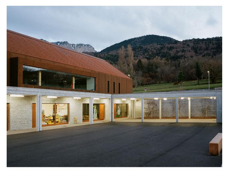
The construction principle is based on a load-bearing concrete structure, framed using pine battens and insulated from the inside. The structure of the refectory is built with timber frame walls for the façades, while the roof frame is in wood. The Corten steel envelope resonates with the existing tile roofs. This structural system and the materials were chosen for their rationality, simplicity of lines, and precision of design, while respecting a tight budget and a limited environmental impact.
