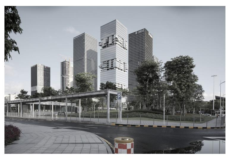
In plan, the tower is a simple square of  $45 \text{ m} \times 45 \text{ m}$ , with 42 floors and an overall height of 200 m, and it features a total floor area of  $80,500 \text{ m}^2$  above ground. A skirt building partially frames the tower at the base, where the entrance area, the public business hall and a high-end restaurant are located.
