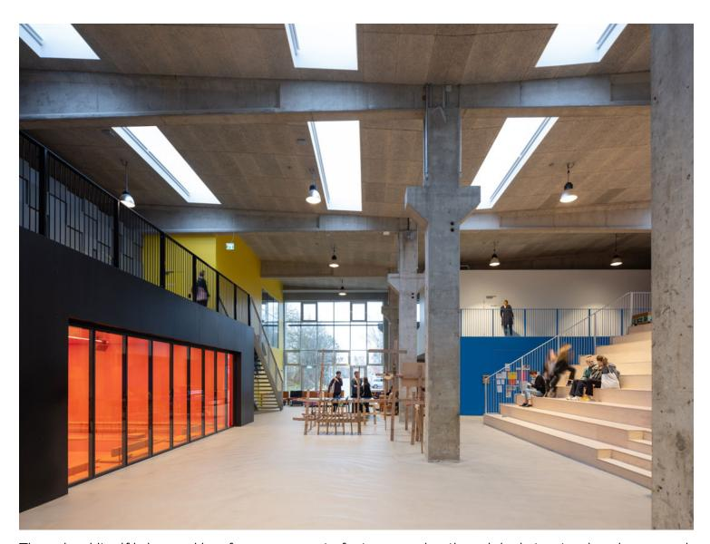
The school itself is housed in a former concrete factory, reusing the original structure's columns and roof but replacing the walls and interior. The design is based on a "box-in-a-box" concept: colorful modules fill the warehouse-like shell of the main building, all arranged around a central spine cutting from one side of the building to the other. Alongside this route is a wooden tribune that acts as the communal heart of the school.
