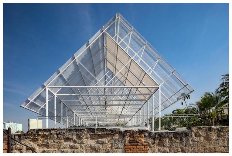
Light and industrialized synthetic materials such as the PVC deck, polycarbonate sheets, and railings made of nylon nets seek to reduce the weight of the construction and generate a strong contrast with the materiality of the historic building. Two different types of polycarbonate were used (translucent and transparent) to filter the sunlight, while maintaining views of the sky from the courtyards.
