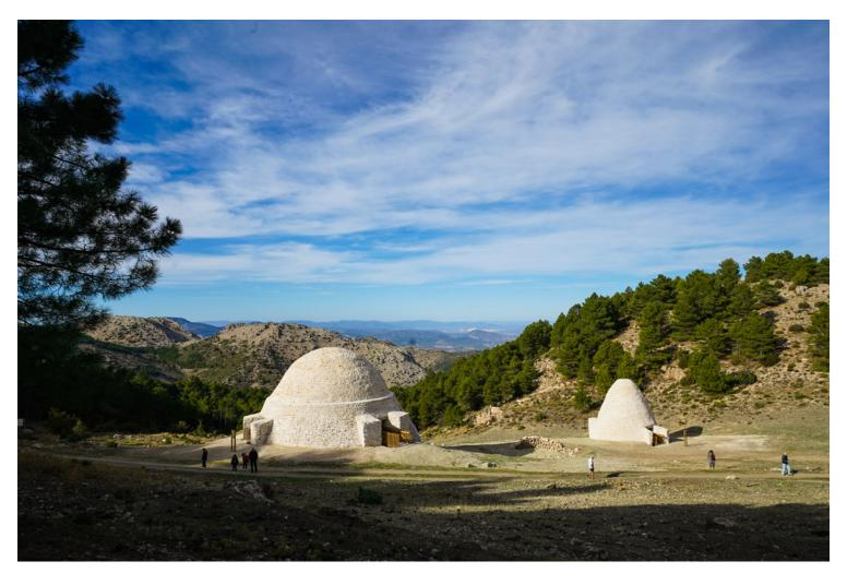
Among the urgent measures outlined in the Master Plan was the restoration of wells number 11 and 13 due to their uniqueness, accessibility, and state of conservation. Despite significant damage and the collapse of a substantial part of their domes, they still retained enough structure and data for their recovery.
