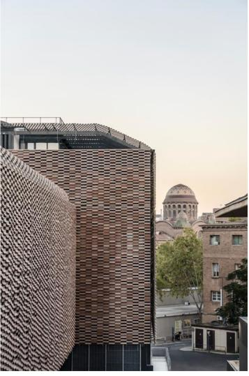
The façade is simple and efficient, making use of sandwich panels with good insulation. These panels are protected by a technological ceramic skin as a latticework, with the same chromatic range as the historic pavilions of the *Modernista* hospital. This skin ensures a drastic reduction in energy demand (in a building with very significant internal thermal loads). In turn, it allows for the entry of natural light, while providing views to the outside and guaranteeing researchers' privacy.
