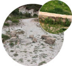
STONES FROM ROCKFALLS TO BUILD THE RETAINING WALLS
