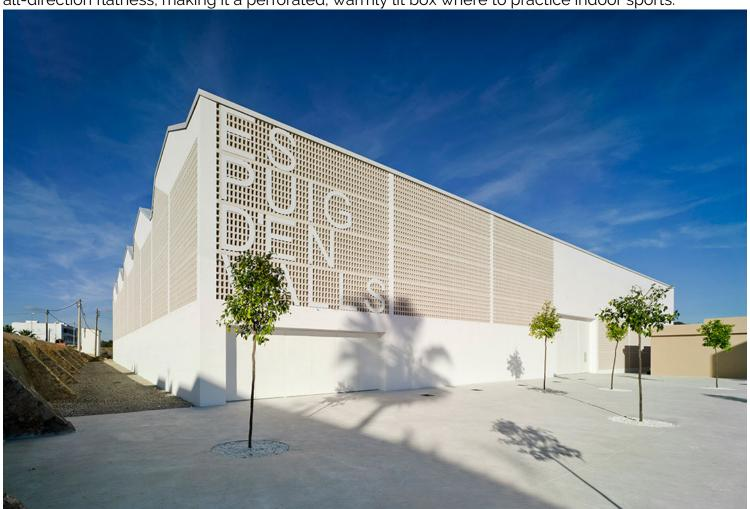
The project for the EsPuig d'en Valls Sports Centre was conceived in two distinct phases: the first consisted of covering the two existing outdoor courts; the second was the design and execution of the perimeter enclosure.
